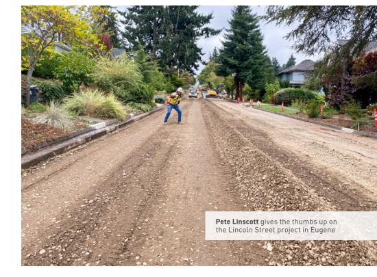
of general excavation for installation of new asphalt and concrete roadways. To date this team has installed 2,900LF of storm and sewer pipe, 36 inlet structures, 16 manhole structures, 31 ADA Ramps 4,500SF of sidewalk, 1,800LF of curb and gutter. In addition, 3,000TN of aggregate base was placed for 1,700TN of asphalt paving in late October.
